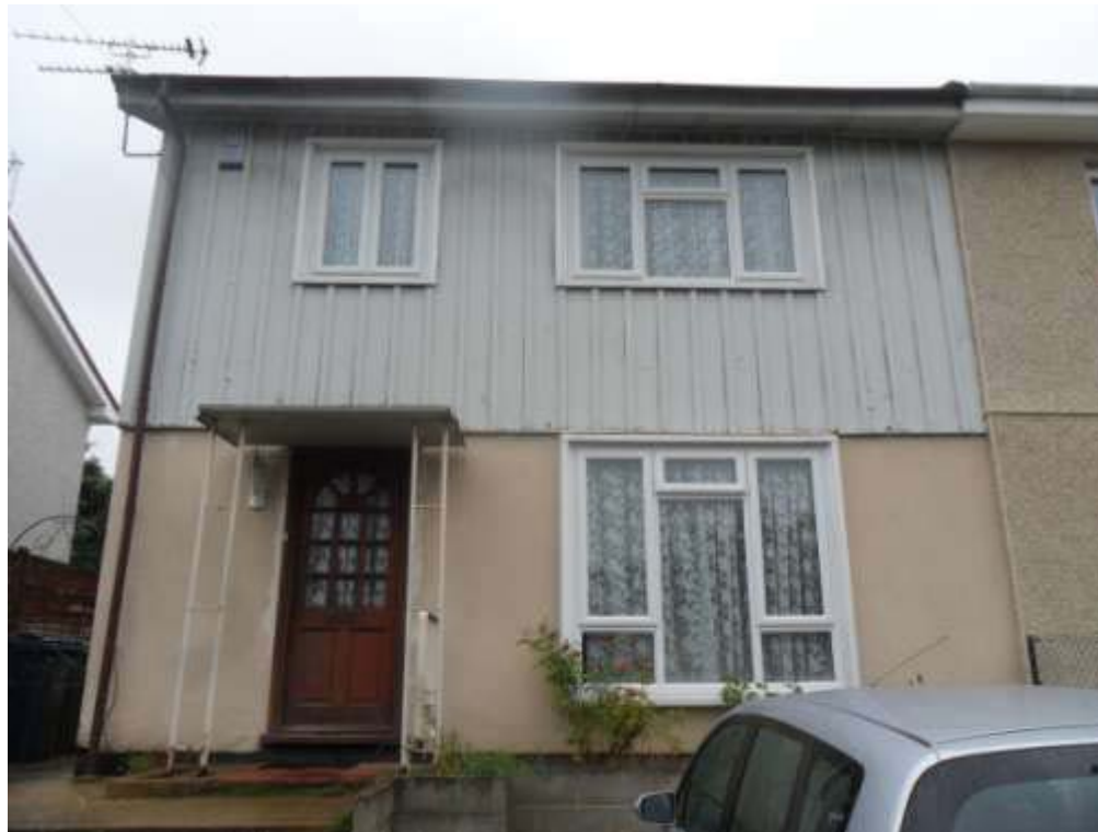
TYPICAL EXISTING HOUSE
