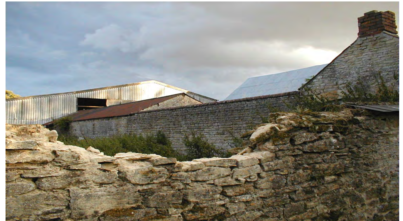
Existing stables from the north west
