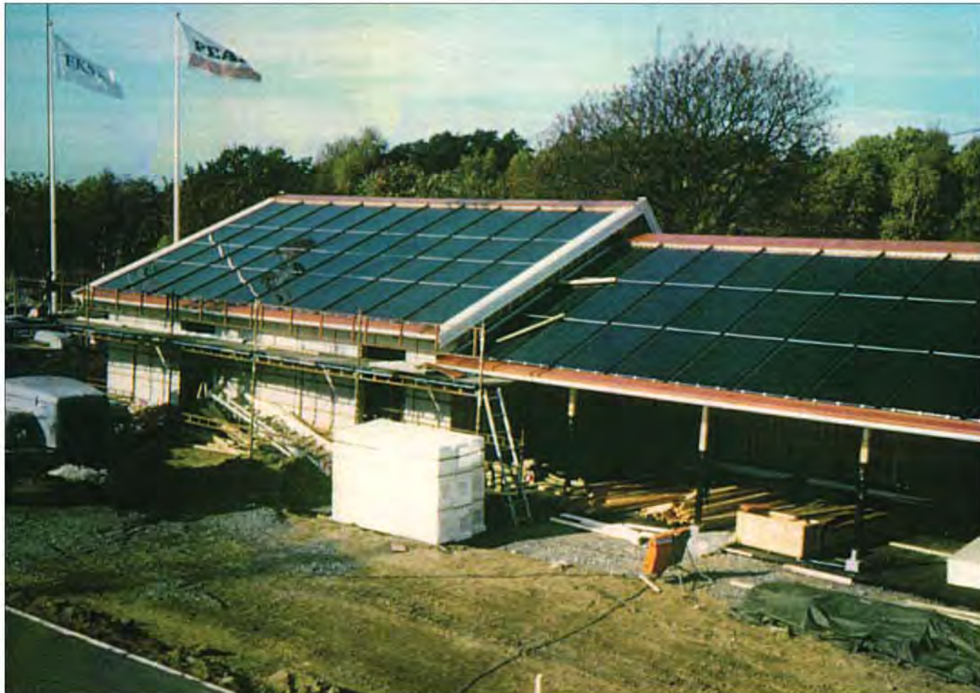
Installing the roof module collectors at Onsala, Sweden.
